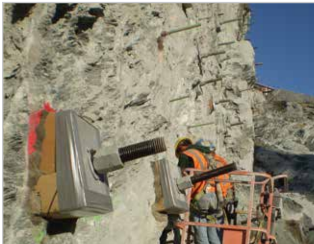
Anchors stabilize the rock face of the Holtwood Dam.
