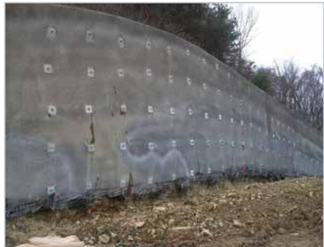
Soil nails used at the Moretrench Avonworth Primary Center
