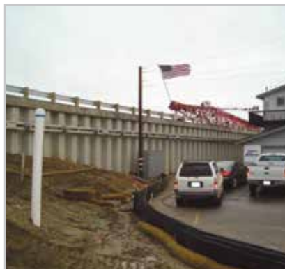
Stage 2: Soil is placed between the two walls and compacted.
