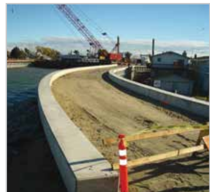
Stage 3: The structure is able to carry vertical loads as well as provide flood protection.
