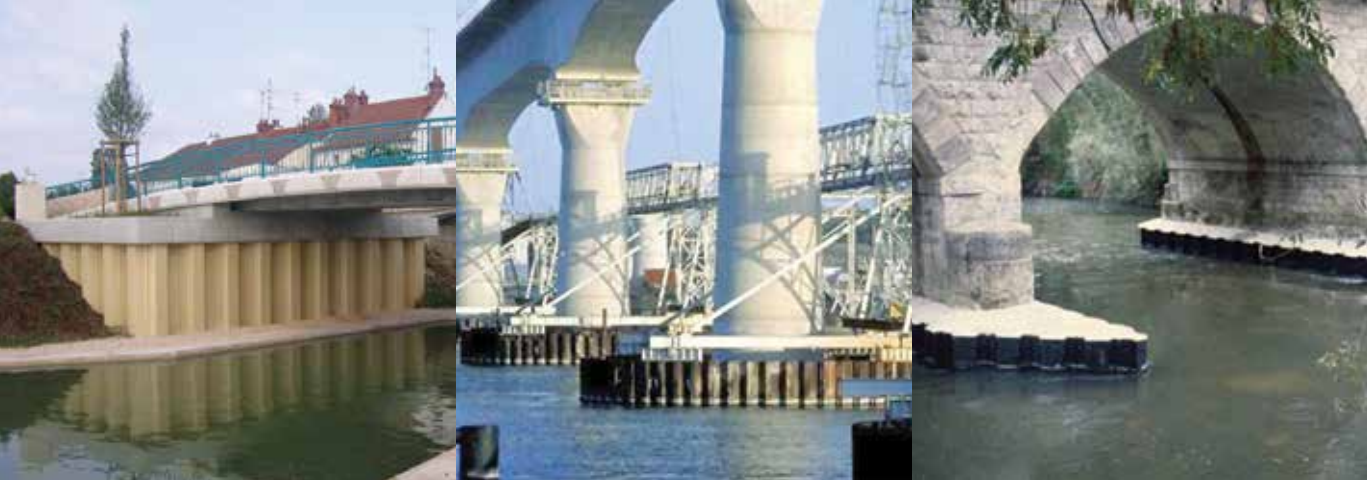
Permanent steel sheet piles protecting bridge abutments and piers from scour related problems.
