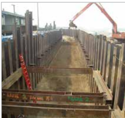
Stage 1: Parallel Z-type sheet piles are installed and tied together with a threaded bar.
